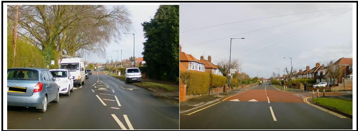
View heading east to school access Fulfordgate raised platform.
